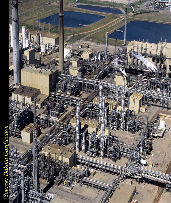
Pre-Combustion Capture (coal gasification plant, USA)
