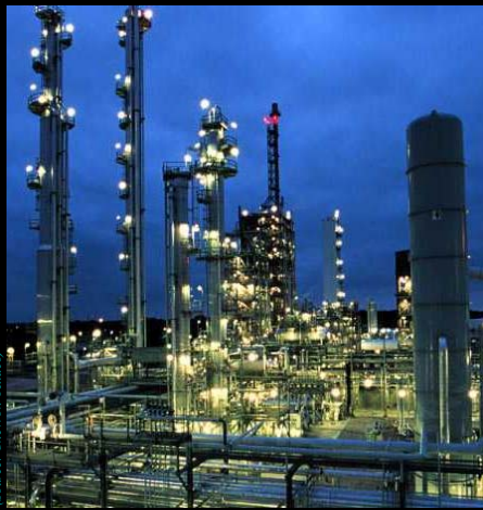
Petcoke Gasification to Produce H 2 (Coffeyville, Kansas, USA)
